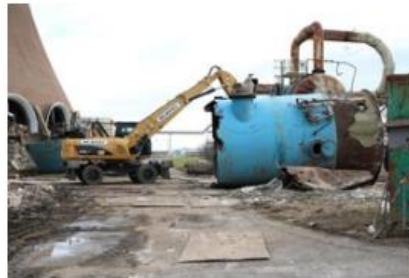
Decommissioning has begun at Olefins
