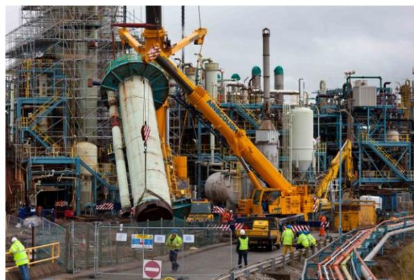
Since the sequential decommissioning and demolition of five redundant chemical processing plants began on the high-hazard Runcorn site in August 2010, the site remained operational elsewhere. Meticulous planning and project coordination was therefore essential to ensure minimal disruption and utmost safety for all parties.
