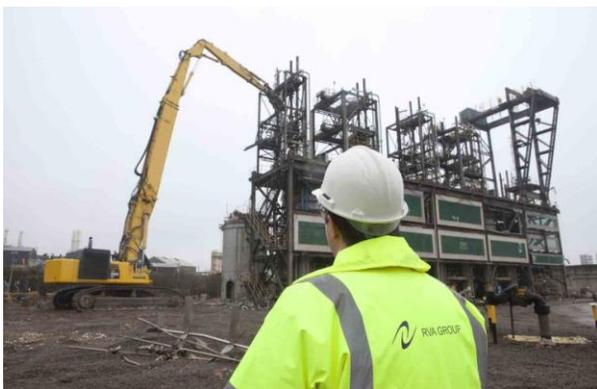
Utilising its vast knowledge and experience of asset recovery, RVA recommended that INEOS hand the site back as flat slab, as plant demolition and dismantling could generate an income from the sale of the process equipment – some had potential for reuse whereas other items (as a result of their high-value metallurgy) would create a positive income stream.
